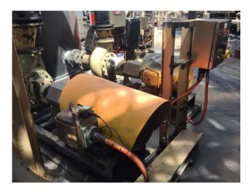
The above application shows the K-MotorShield Motor Cover being used on pumps to ensure they stay unaffected by the fine powder covering the site.
