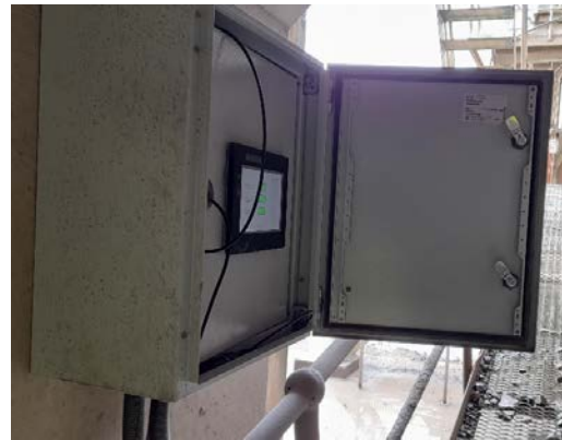
Figure 30 - Control box for live data view and logging
