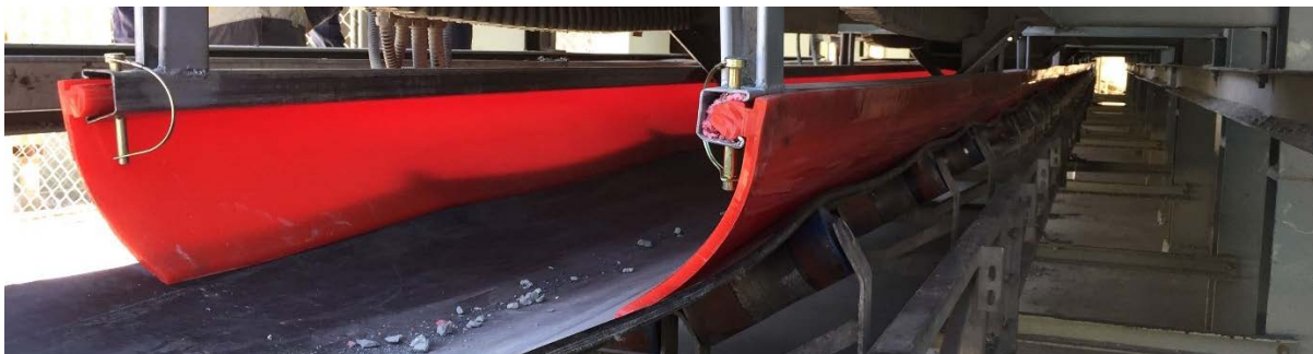
Figure 10 - K-Snap Loc® lay in belt skirting system can self-adjust to belt sag and skirting wear
