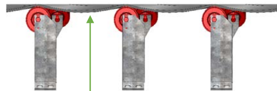
Belt sag due to lack of support
