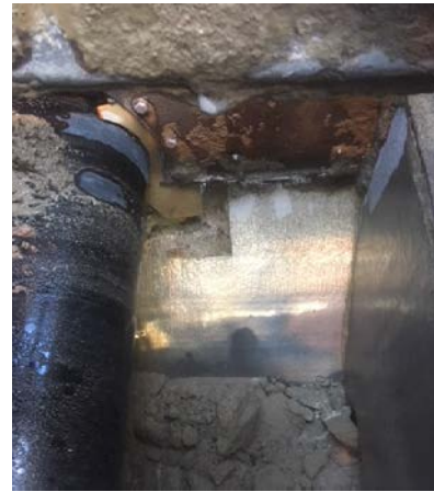
Recycling Pugmill – After Installation
