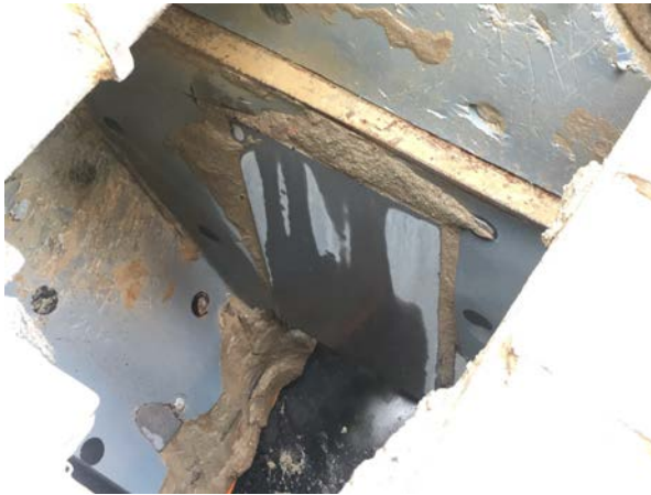
Recycling Pugmill – Before Installation
