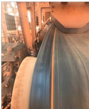
Photo: Typical groove caused by product build-up in skirted section.
