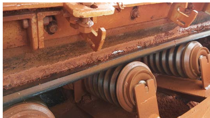
Photo: Typical product build up behind hardskirt.
