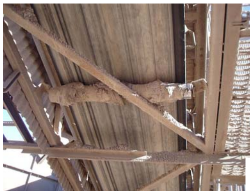
Right: Typical return roller clogged with wet conveyed material, creating a build up of spillage, and long term potential to damage the belt itself.
