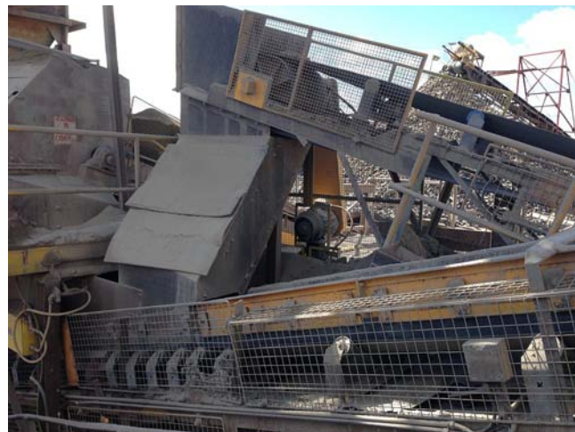
Right: photo showing the site's conveyor height and transfer chute angle on the way to the crusher.
