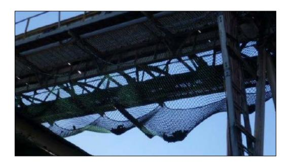
Workplace safety, hazard identification and prevention steps require careful consideration. Falling objects such as debris, rocks, other large conveyed materials as well as conveyor rollers during routine replacement can cause serious injury to workers and costly damage to property.
