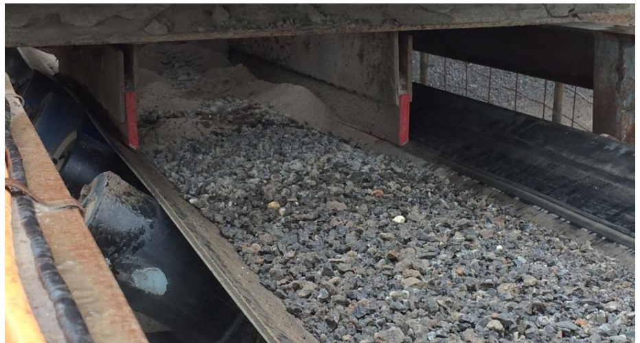
Close-up photo of the K-Superskirt® Engineered Polyurethane installed on one of the conveyors at the transfer point.
