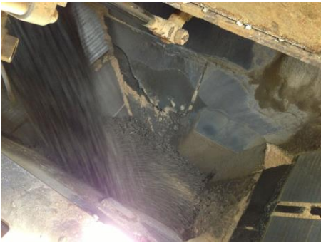
Photo of the internal sides of the hopper, showing the worn and uneven surface.
