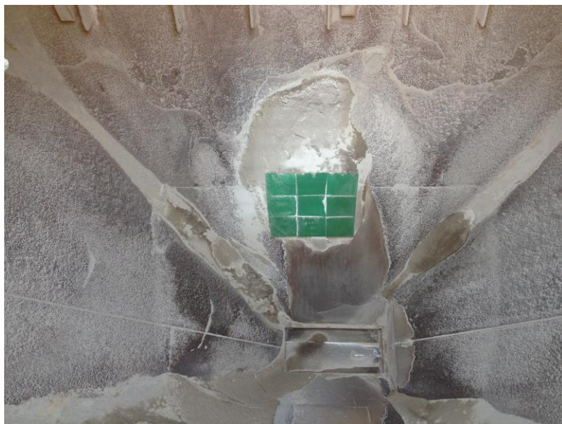
K-Redi-Liner® Polyurethane in place at bottom of the chute of St Peters rail terminal
