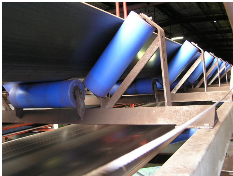
Photo taken of K-Polymer Conveyor Rollers on site at Yallourn Power Station.
