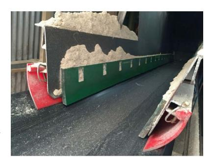
Photo showing the combined installation of K-Containment Seal with the height adjustable slots, together with the simple unistrut mounted K-Snap-Loc®.
